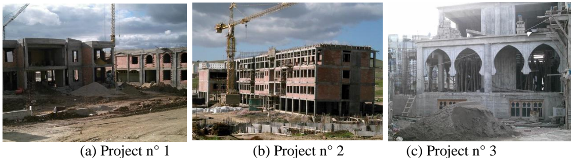
Figure 1. Overall view of the projects
